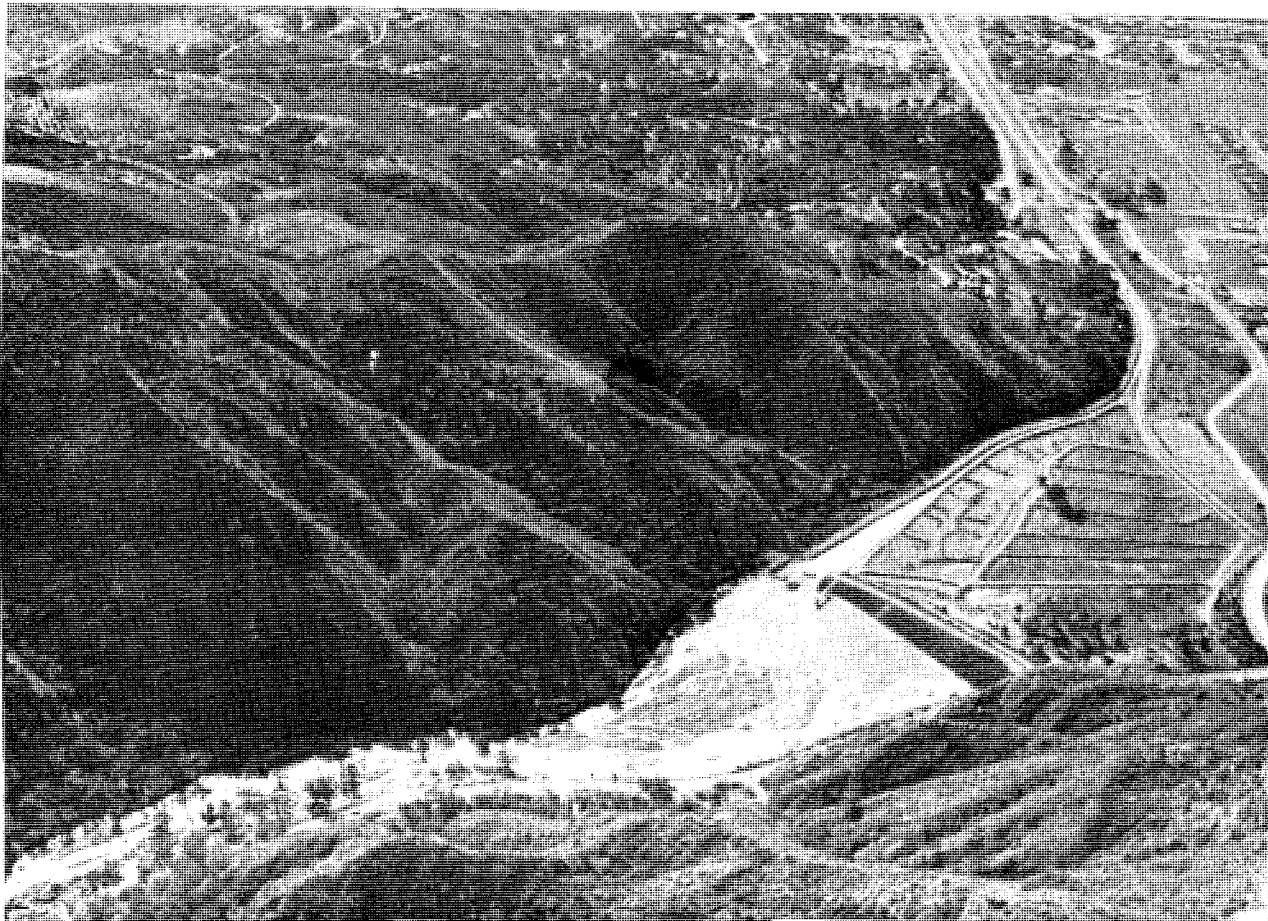
Big Dalton Debris Basin
